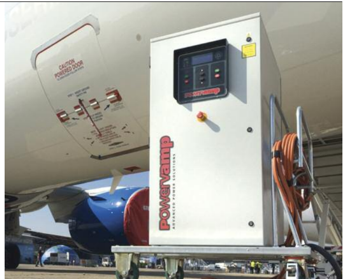
PV90-3: specified to provide ground power at the Paris International Airshow 2017
