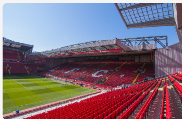
EF 33 ELI (120kVA) installation at Anfield Stadium, Liverpool
