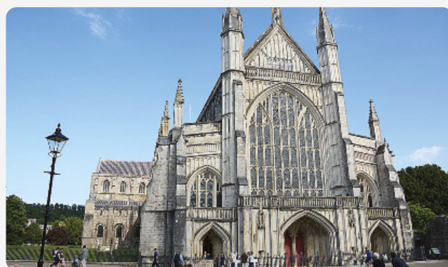
EF5 x 4 (300VA - 600VA) installations at Winchester Cathedral
